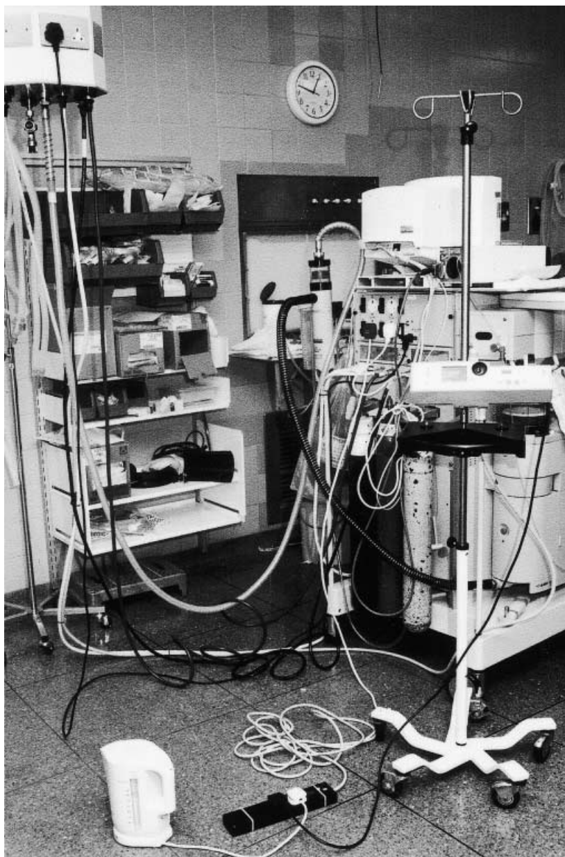
Figure 1 Arrangement of electrical components involved in the incident.
