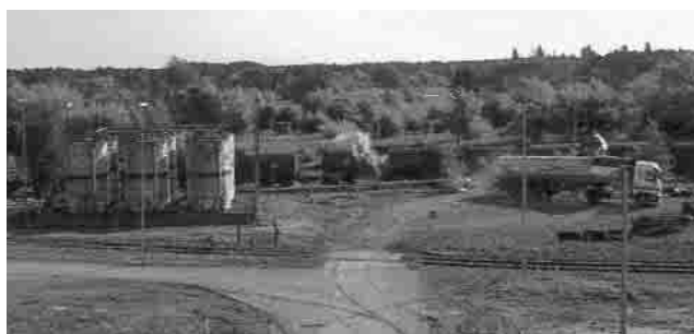
Fig. 13 – Un-loading of heavy oil and animal fat feeder tanks of the oil injection facility.
