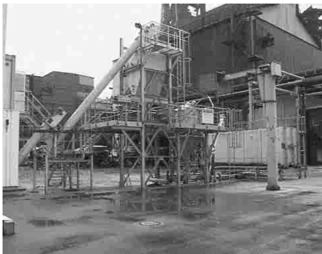
Fig. 7 – Plastics unloading station, coarse grain segregation.
